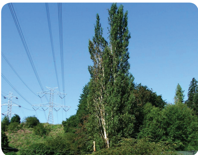
Trees that grow too close to high-voltage power lines are a hazard. In certain circumstances, electricity can jump or arc from the lines to the trees, which can cause power outages, fires and serious injuries to anyone near the trees.
